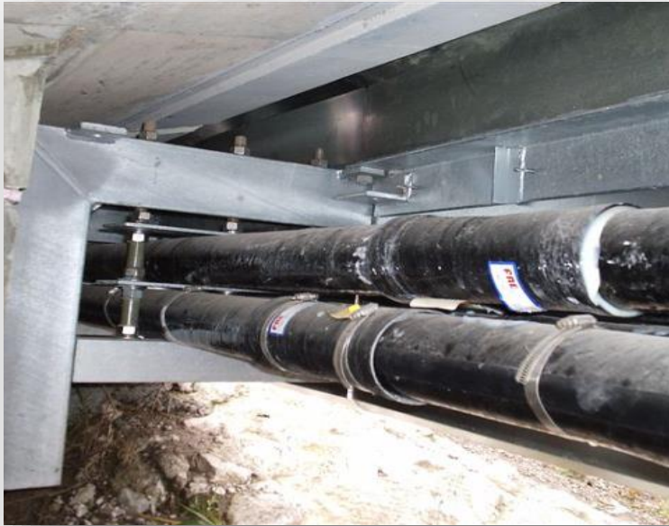
Duct hangers & brackets
